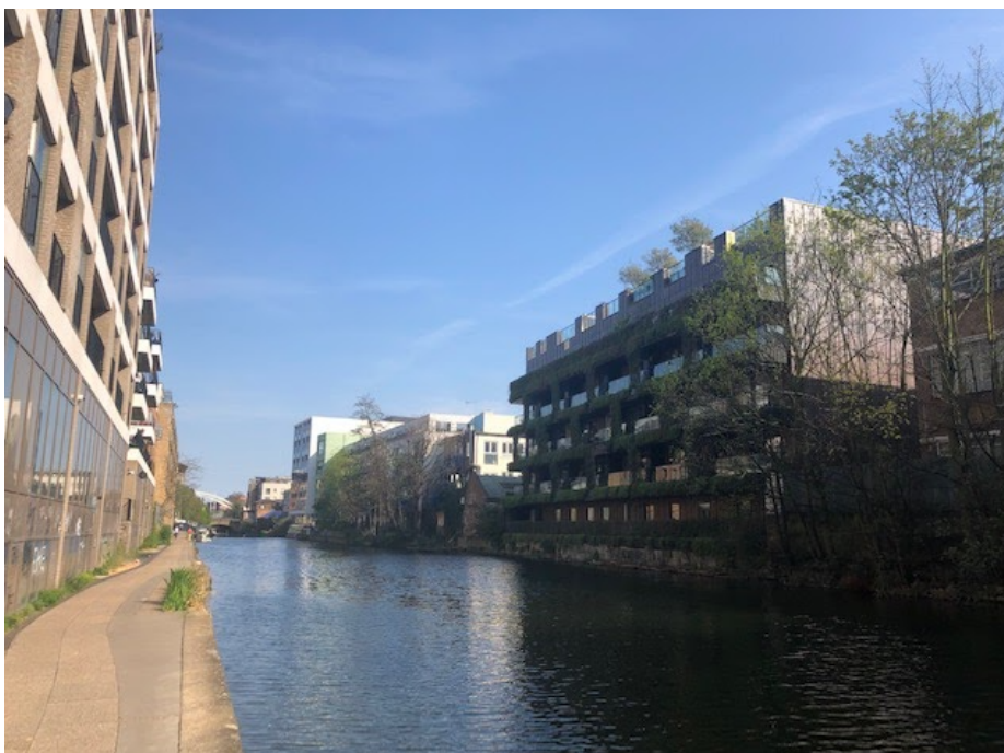
Canal context showing existing buildings
